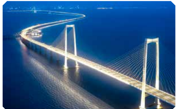
► Shenzhen-Zhongshan Corridor Lighting Project
