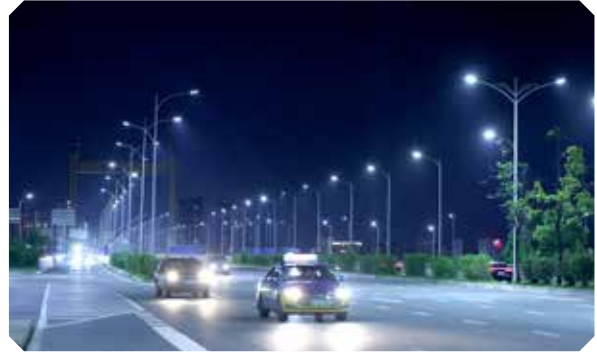
► Fuzhou Urban Road Lighting Project
